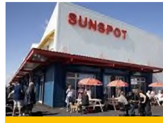
Solar panels to Sunspot
